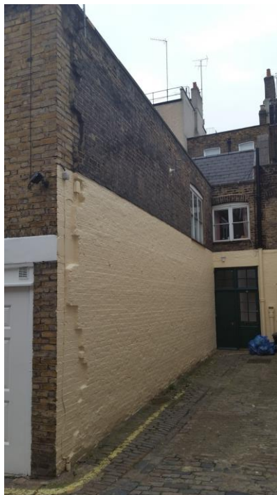
North elevation, facing Wigmore Place
