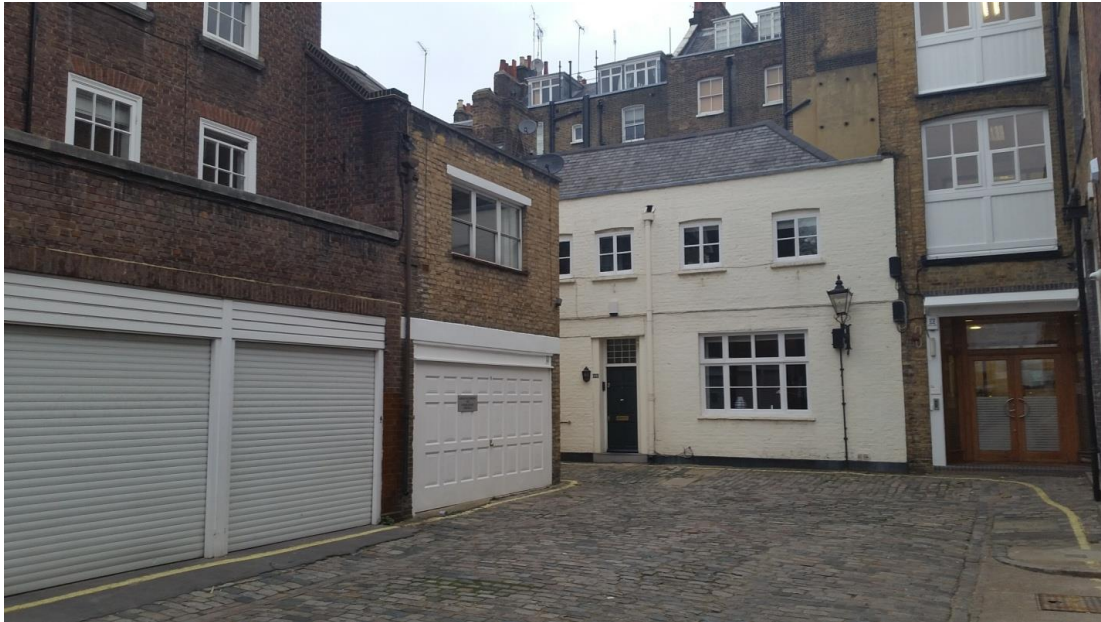
West elevation, facing Wigmore Place
